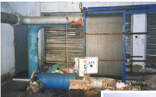
Bernoulli Filters protect plate heat exchangers in a power plant built by Sulzer.
