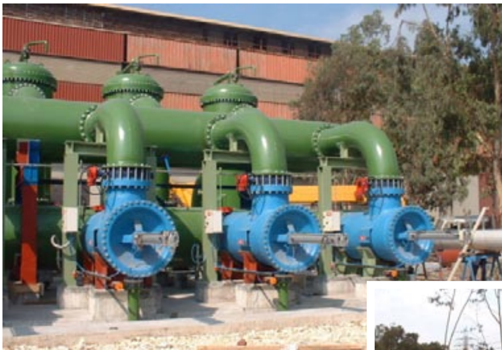
Bernoulli Filters protecting the cooling system in a steel works.
