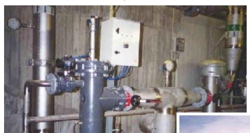
Unmanned power stations need reliable, maintenance-free equipment. Graningeverken chose Bernoulli Filters as intake water filters for generator and bearing cooling at the Degerforsens plant in Junsele.
